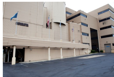
The plant was designed to look like an office building in order to help it blend into its surroundings.
